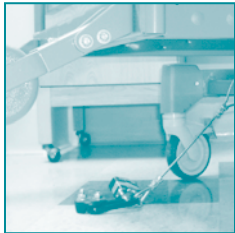
Bed is anchored and locked to the floor to prevent barricade situation. This is thought to be a safety feature.
